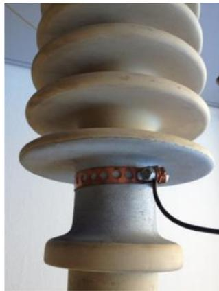
conductive coating might be necessary to create a good conductive band for the leakage current to choose the path through the LC-Track rather than directly down to earth. Make sure that the connection onto the insulator provides a good conductive path all around the base.
